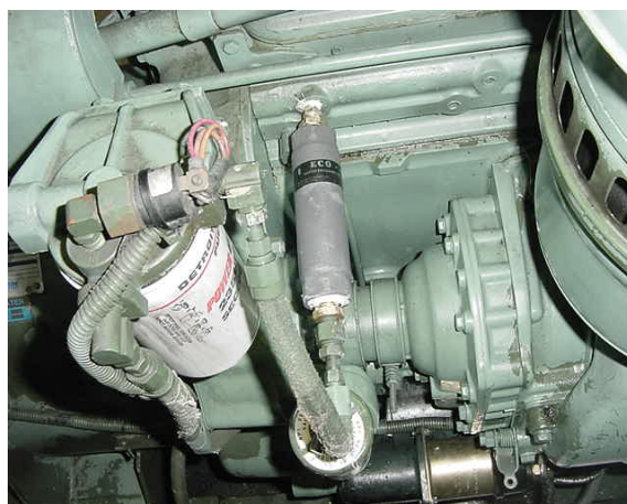
ECO-4 installed on both 471 Detroit Generators
